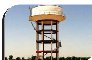
Dedicated Water Tank
